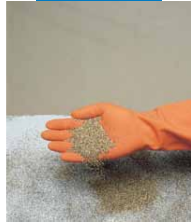
Spreading dry sand on fresh Mapecoat I 24
