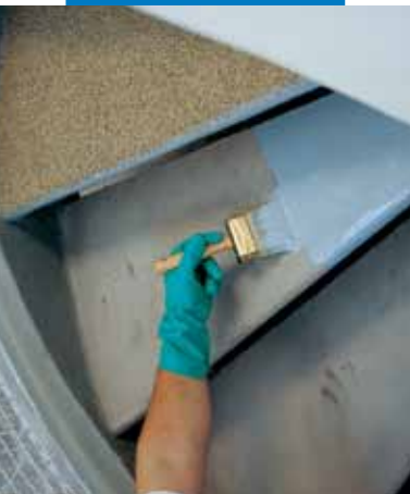
Applying first coat of Mapecoat I 24 on concrete
