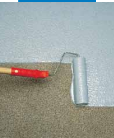
Applying Mapecoat I 24 with roller
