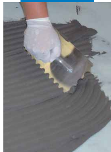
Application of suitable MAPEI tile adhesive over Mapetex
