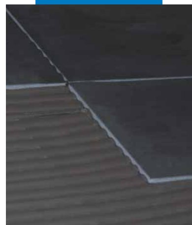
Installation of tiles over Mapetex
