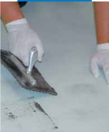
Smoothing Mapetex in place with trowel
