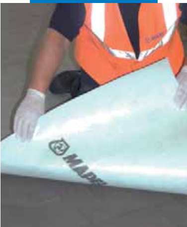
Installation of Mapetex over Keraquick & Latex Plus
