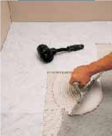
Setting white Carrara with Keraquick white
