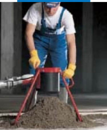
Batching a Topcem mix
