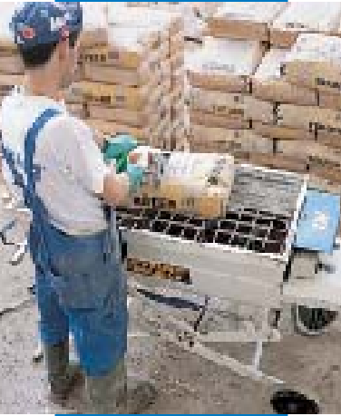
Mixing Topcem in a mini-batcher
