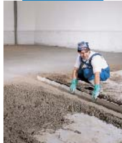
Preparing a levelling strip
