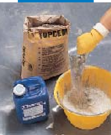
Mixing Topcem with Planicrete to make an anchoring slurry
