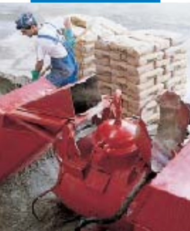
Mixing Topcem with an automatic pumping unit
