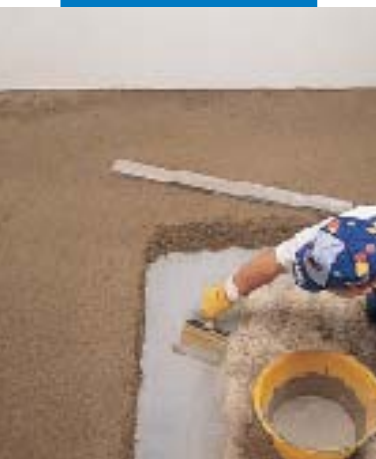
Spreading the anchoring slurry for integral Topcem screeds
