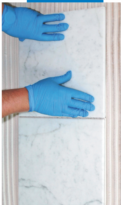
Application of Mapeker Rapid-Set Flex on 15 mm plywood
