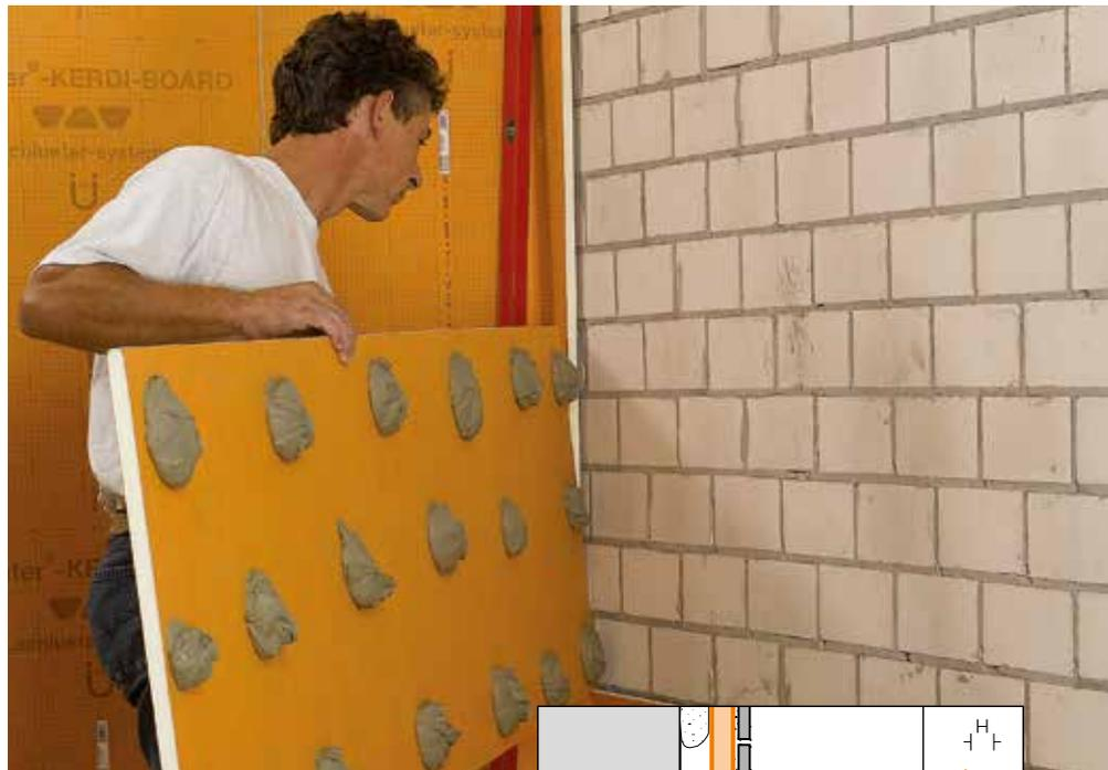
Schlüter®-KERDI-BOARD can be fully adhered in wall areas or alternatively attached with dabs of thin-bed mortar or another suitable adhesive or mortar. If necessary, the material may be secured with additional wall anchors. In the case of stud frames made of wood or metal, Schlüter®-KERDI-BOARD is attached with screws from the matching hardware system.
